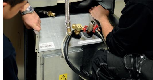
4. Pull the cooling module by first lifting the front edge slightly with the carrying handles.
