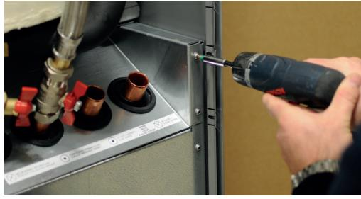
3. Unscrew the cooling module's screws.
