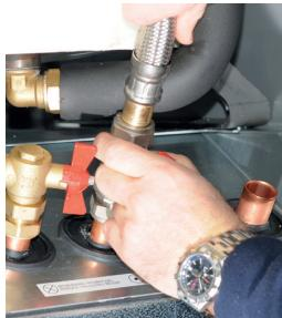
1. Disconnect the cooling module's power cable connector and hoses.
