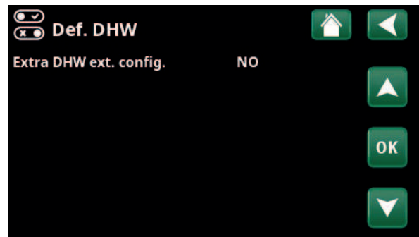
Menu: "Installer/Define/DHW" On menu bar "Extra DHW", the normal mode is specified for the external control signal ("Normally Open (NO)" or "Normally Closed (NC)").
